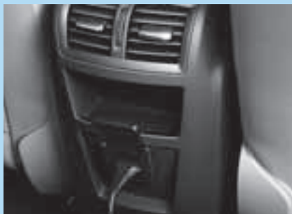
230-volt rear power outlet.
